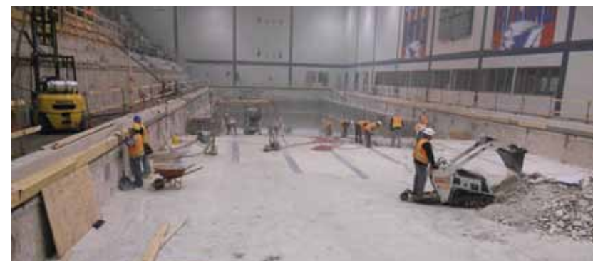
United States Air Force Academy cadet gym modernization project.
