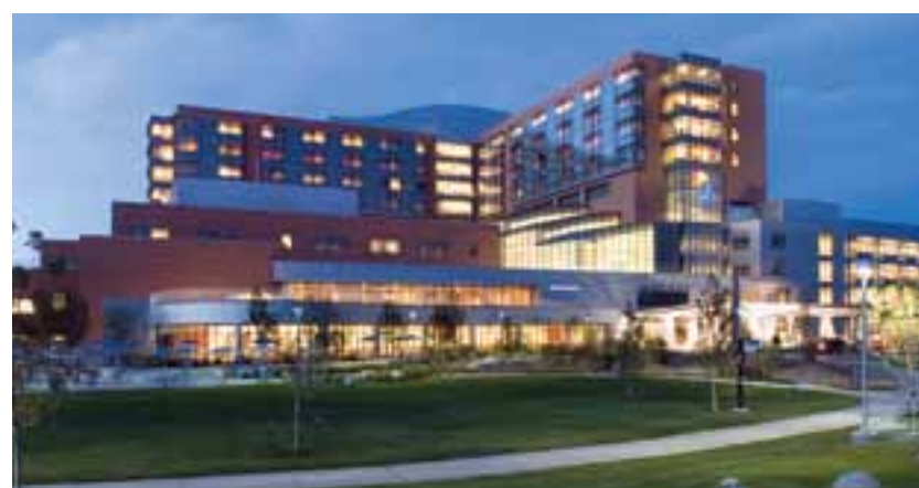
Children’s Hospital Colorado Aurora, Colorado
