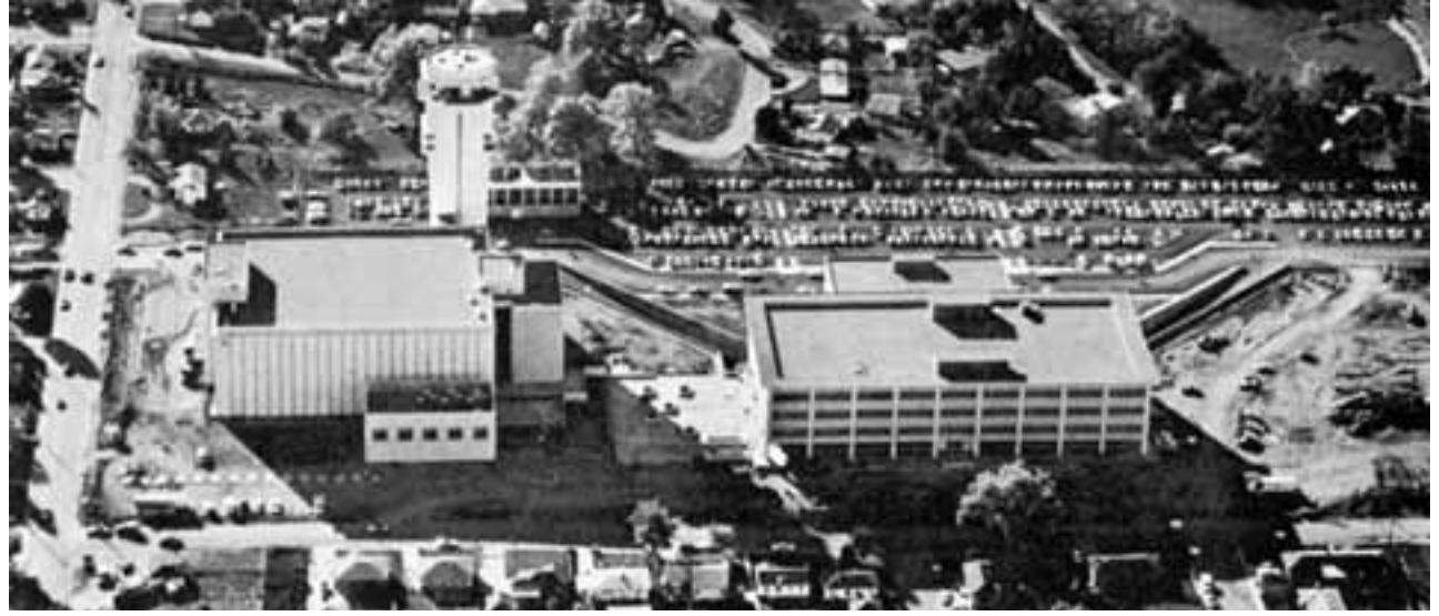
Century Link Zuni Communications Center Denver, Colorado
